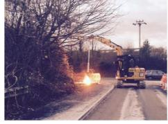
that the base of the column could be slid into the sleeve. As the column was moved towards the vertical position, it came into contact with SSE 11kV overhead cables located directly above the sleeve. This resulted in the ground worker, who was holding the base of the lighting column, receiving an electric shock and contact/exit burns.
